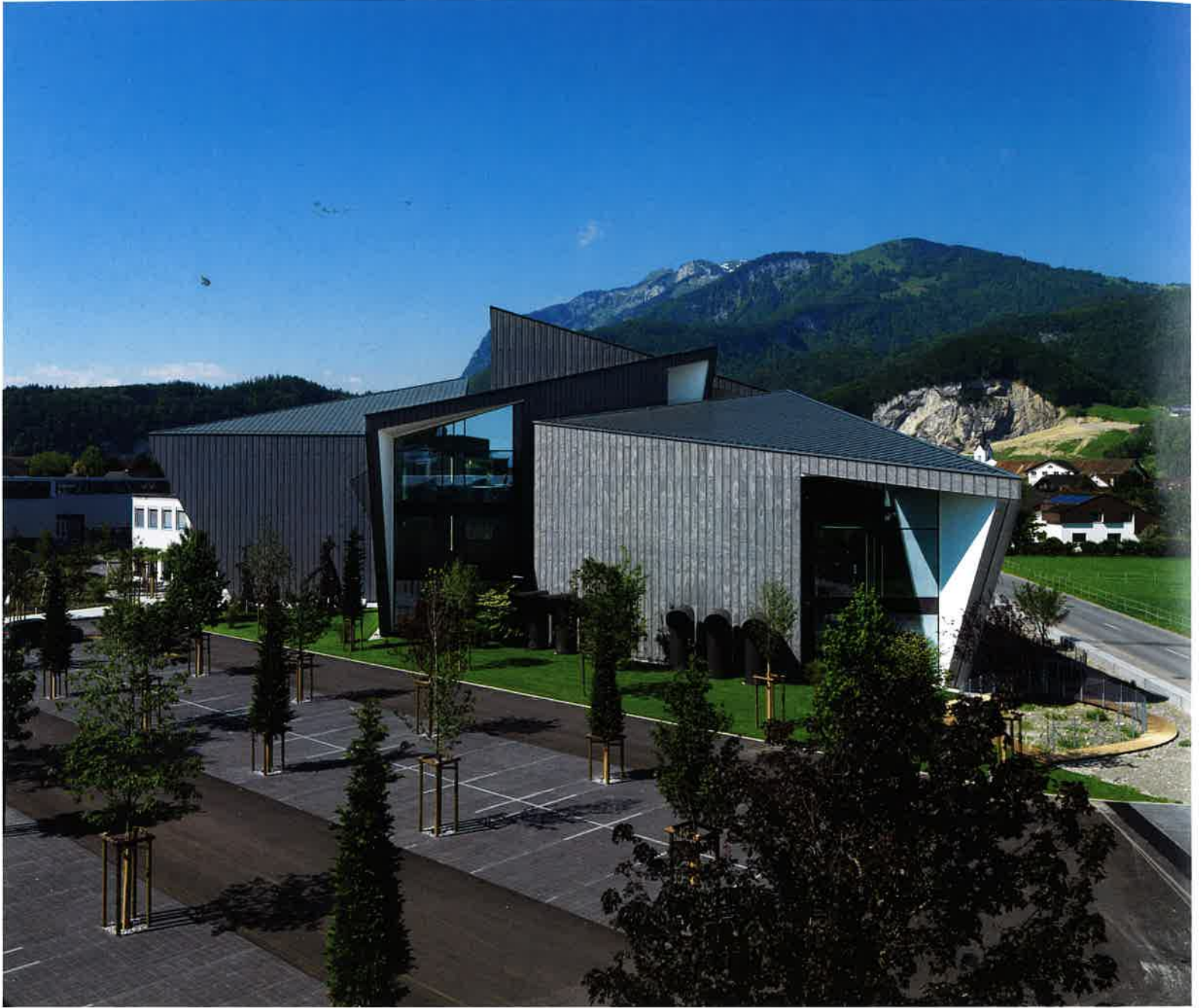
↑ | Façade, clad in a dark perforated zinc mesh → | Night view, pool serves as rainwater collector
