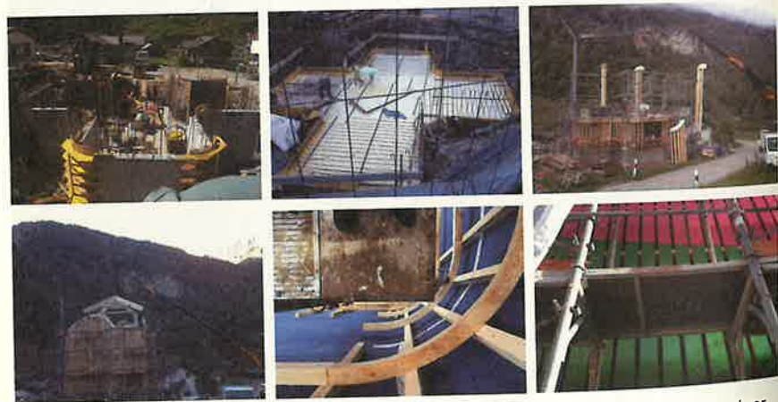
Construction process of Swisshouse XXXII ©Alexandre Zweiger
